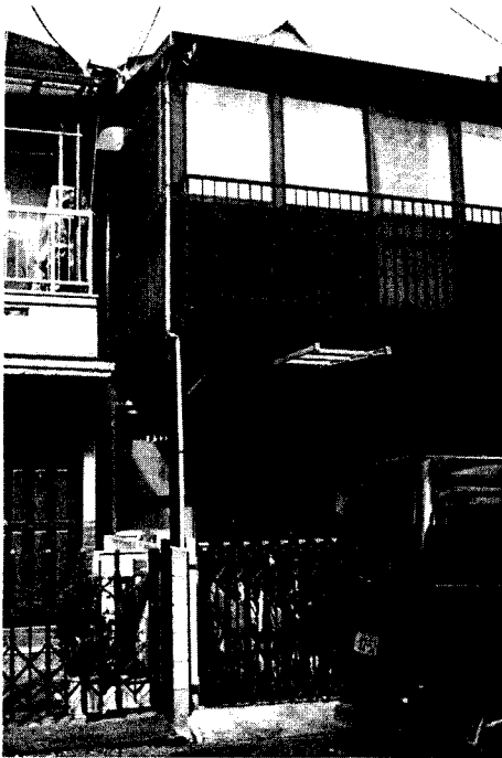
Fig. 6. Typical light-gauge steel framed residential building.
