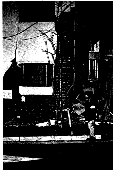
Fig. 10. Latticed beams and columns in three-storey residential building with wood lattice infill (note collapsed first storey).
