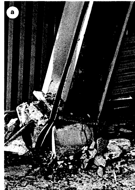
Fig. 38. Damage to column base connections: (a) anchor bolts fractured; (b) anchor bolts pulled out; (c) concrete encased column base rupture. (Courtesy of the Architectural Institute of Japan.)
