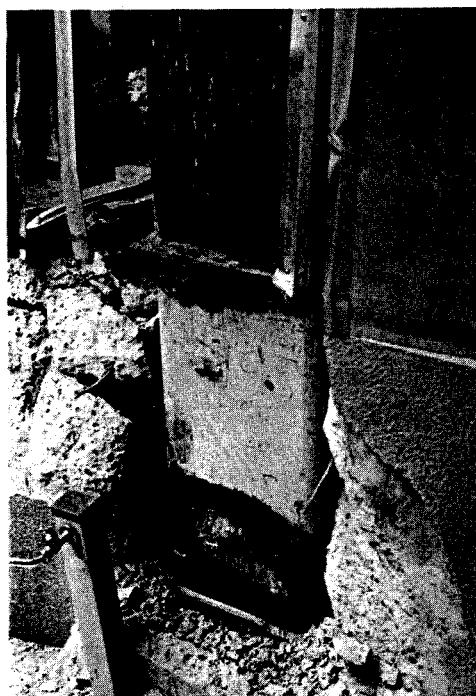
Fig. 35. Column damage in a braced frame.
