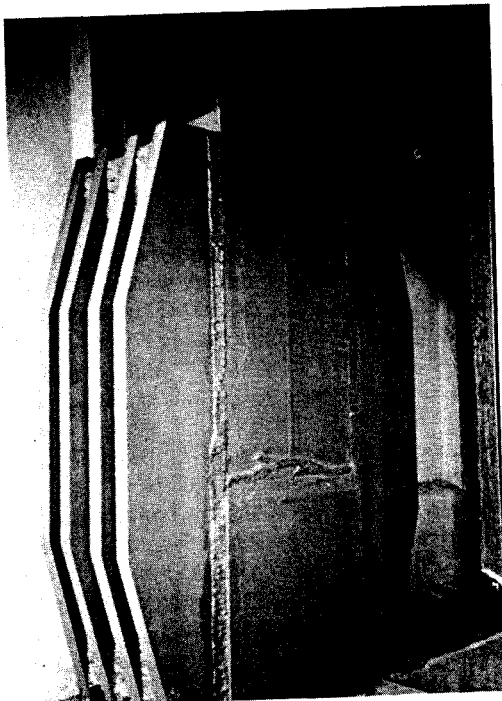
Fig. 41. Welded of and addition of reinforcement plates to cracked columns in the Ashiyahama Residential Complex.
